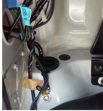
Ground located inside cab, driver's side left kick panel
